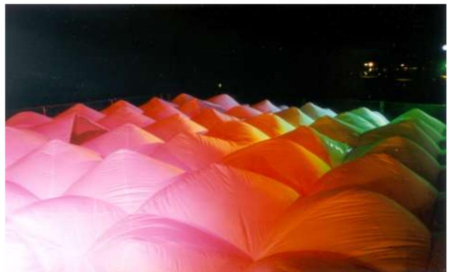
The Space Maker is a tent with an interactive moving roof. The roof is normally too low to stand in the tent. At the places visitors move towards, the tent roof rises up automatically so you can stand there. When you walk, ahead of you the roof goes up, and behind you it goes back down. That way, the volume of the tent stays minimal.
