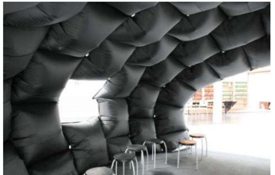
Inflatable folly for in- and outdoor video presentations. The folly creates a separated dark space in a larger environment. The construction consists of connected individual airbags. The different shaped bags and the pressurized air inside give the tent its shape and firmness. The construction leans against the wall which can be used as a projection screen.
